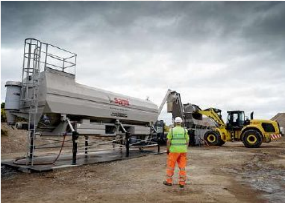
Pat Munro's mobile batching plant and silo at Dornoch Quarry.
